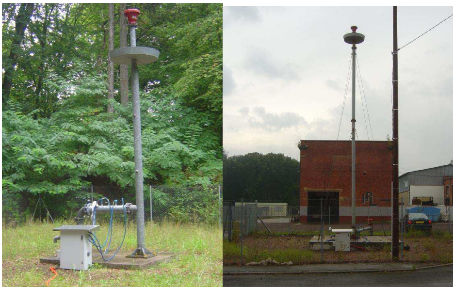
Fig. 1 Photographs of the venting borehole SDEC OUEST 1 (left) and Barrois shaft with a vent (right) (Lorraine coal basin)
