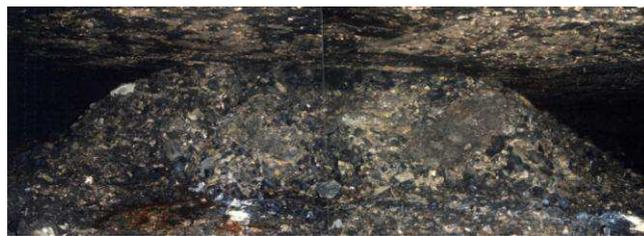
Figure 1: Photograph of a collapsed coal pillar.
