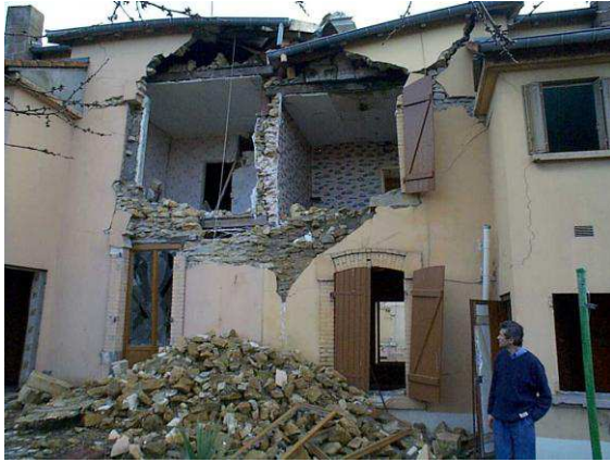
Figure 3. Effect of severe subsidence in Lorraine iron field (left) and major collapse of a chalk mine (right).
