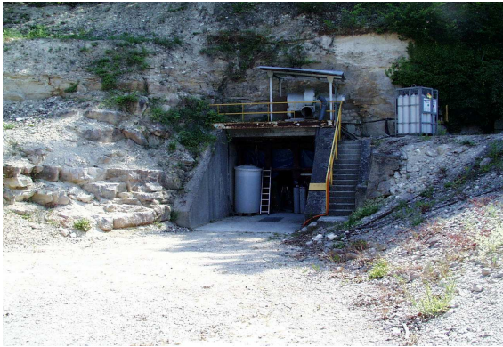
Figure 1: General view of the experimental set up environment
