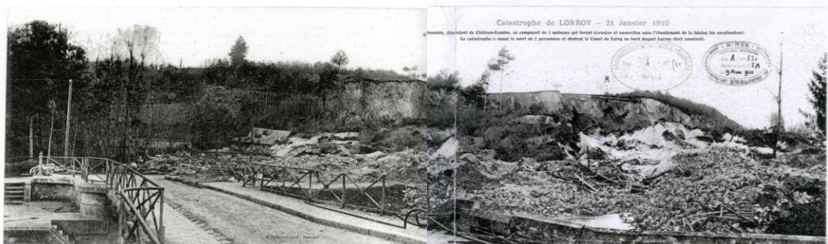
Figure 5: View of the Lorroy site after the disaster of the chalk mine collapse.
