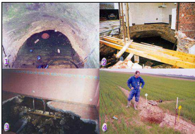
Figure 3: (1) Flooded cellar; (2 & 3) Collapses of buildings due to undermining cavity failure; (4) Backfill run out of an old chalk mine.
