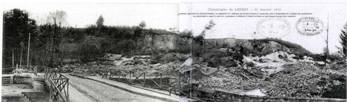
Figure 5: View of the Lorroy site after the disaster of the chalk mine collapse.
