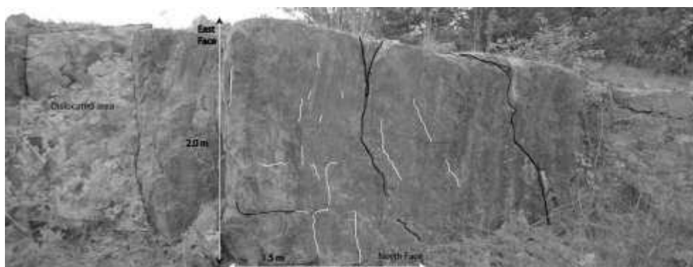
Figure 17: View of the rock mass, it presents a dislocated area on the left, and major discontinuities are in black and superficial are in white.
