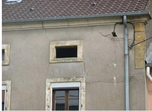
Figure 4. Example of limited damage incurred following the subsidence in Rochonvillers (Roc\_2008)
