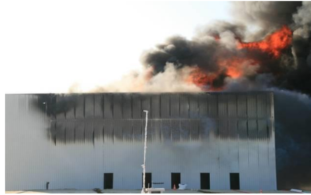
18 min after ignition : roof starts collapsing
