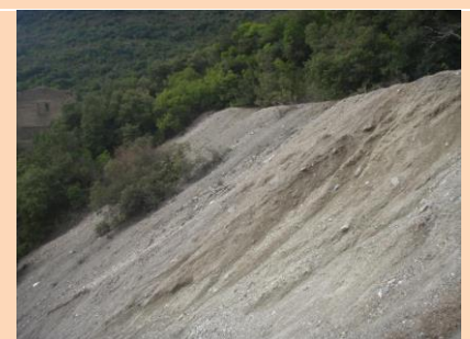
Figure 6 Superficial landslide on a tailing
