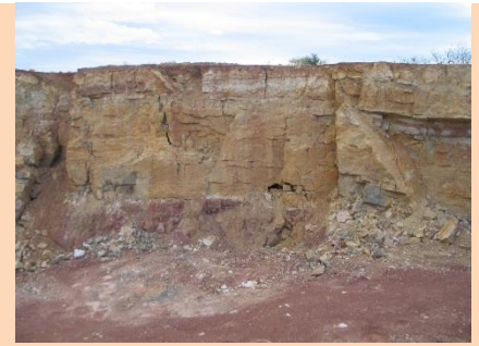
Figure 7 Rockfalls, bauxite mine
