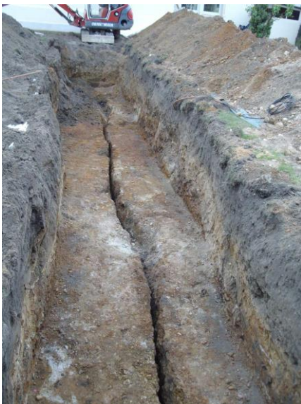
Figure 1. Photograph of a fracture discovered close to the surface (GEODERIS, unpubl.).
